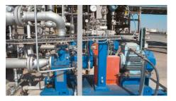
De-ethanizer pump in a LPG fractionation unit of ENOC refinery, **U.A.E.** equipped with an unpressurized dual EagleBurgmann sealing system acc. to API 682. Configuration: 2CW-CS, piping plans 14 and 76. Operating conditions:  $p = 36 \dots 39$  bar (522 ... 566 PSI),  $t = 1 \ ^{\circ}C \dots 43 \ ^{\circ}C (34 \ ^{\circ}F \dots 109 \ ^{\circ}F),$  $n = 2,933 \ min^{-1}$ . Medium: LPG. Since installation, MTBF improved drastically.
