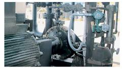
To convey sour water with high SO<sub>2</sub> content, a Weir pump is installed in the fluid catalytic cracker (FCC) of the Amuay-Cardón refinery in **Venezuela**. The shaft is sealed by dual pressurized EagleBurgmann API type A seals and equipped with a barrier fluid system with bladder accumulator. Configuration 3CW-BB, piping plans 02 and 53B. Operating conditions: p = 15 bar (218 PSI), t = 50 °C (122 °F), n = 3,600 min<sup>-1</sup>.
