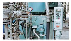
In the Toa Oil FCC Plant in **Japan** the Sundyne API 610 type OH6 reactor recycle pump handling Butane is operating successfully with a dual pressurized face-to-back EagleBurgmann API 682 type A pusher seal. It runs with plans 13 / 54 at 20.000 min<sup>-1</sup> at a sealing pressure of over 66 bar (957 PSI).
