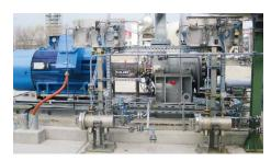
A Sulzer HDS feed pump type GSG 100-300 is applied at Total Refinery in Leuna, **Germany**. Sealed by an EagleBurgmann API balanced pusher seal with containment seal (configuration 2CW-CS). Piping plan 75 (EagleBurgmann gas supply and leakage collection systems).
