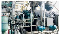
In the Refinery Complex Amuay-Cardón run by Petróleos de **Venezuela**, S.A. our seals are installed in about 90 of the most demanding services. In one of the critical applications, the BB5 Pacific pumps are successfully sealed with dual EagleBurgmann API type A seals and appropriate supply systems. Configuration 3CW-BB, piping plans 02 and 53B. Operating conditions: p = 18 bar (261 PSI), t = 200 °C (392 °F), n = 3,600 min<sup>-1</sup>. Media: Naphtha and Gasoil (3 % H<sub>2</sub>S).
