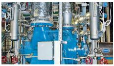
Since commissioning in January 2009, one of the critical pumps in the Bangchak refinery, Bangkok, **Thailand** performes well with a dual EagleBurgmann API type C metal bellows seal with an unpressurized buffer fluid system. Configuration: 2CW-CW, pipings plans 23, 52. Operating conditions:  $p = 1.6 \dots 5.6$  barg (23.2  $\dots$  81.2 PSIG), t = 302 °C (576 °F), n = 1,470 min<sup>-1</sup>. Medium: High temperature hydrocarbon.
