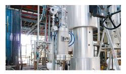
Thompson Byron Jackson cold service pumps circulate light hydrocarbons in the Santos Moomba gas plant in **Australia**. Reliably sealed by EagleBurgmann dual pressurized API type A seals, supplied by a Plan 53C barrier fluid system (max. 40 bar (580 PSI)). Configuration 3CW-BB, piping plans 53C and 61. Seal pressure: 10% above discharge pressure (32 bar (464 PSI)), t = -20 °C ... +38 °C (-4 °F ... +100 °F), n = 1,480 min<sup>-1</sup>.
