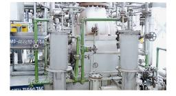
A dual EagleBurgmann API type C double ply bellows seal performs well in a Kirloskar Ebara debutanizer reboiler pump which is installed in the RPL refinery complex in Jamnagar, **India**. Configuration: 2CW-CW, piping plans 21, 52. Shaft diameter: 130 mm (5.12"). Operating conditions:
