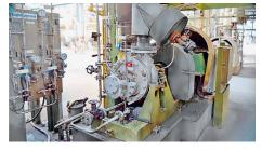
In the naphta processing of a refinery in **Germany**, a 4 ROV 2-stage pump (Ruhrpumpen) is sealed with EagleBurgmann API type A dual pressurized pusher seals. Configuration 3CW-BB, piping plans 53B + 62 (nitrogen).
