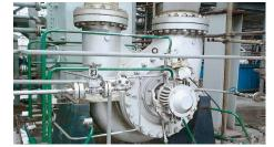
Fujian Refining & Petrochemical Co., Ltd. in **China** applies a BB2 pump for propane de-asphalting. The shaft seal is an EagleBurgmann API type A seal. Configuration 2CW-CW, piping plans 21+52. Operating conditions: p = 73 barg (1,059 PSIG), t = 165 °C (329 °F), n = 2,970 min<sup>-1</sup>.
