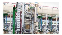
PTT Phenol in Rayong, **Thailand**, operates in its plant a vertically suspended double-casing volute pump. It is sealed with an unpressurized dual EagleBurgmann API type A seal. Although the application is most critical, the seal performs well since May 2008. Configuration: 2CW-CW, piping plans 11 + 52. Operating conditions: p = ... 20 barg (290 PSIG),  $t = 15 \ ^{\circ}C ... 40 \ ^{\circ}C (59 \ ^{\circ}F ... 104 \ ^{\circ}F),$  $n = 2,930 \ min^{-1}$ . Medium: Propylene.
